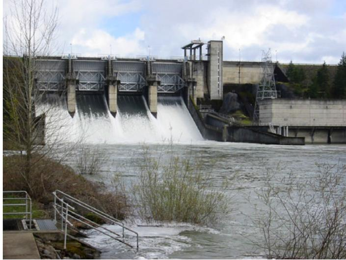
**Figure 1 Foster dam spilling under tainter gates**
