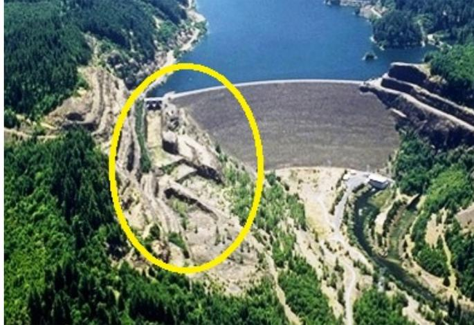
Figure 2 Rocky spillway at Cougar (unsuitable for fish in current configuration)
