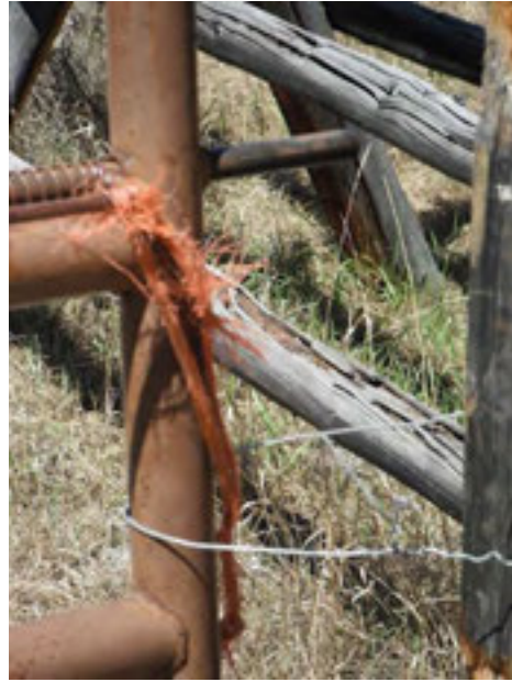
Fig. 1: Closure mechanism of West Fork gate. August 2, 2012.
