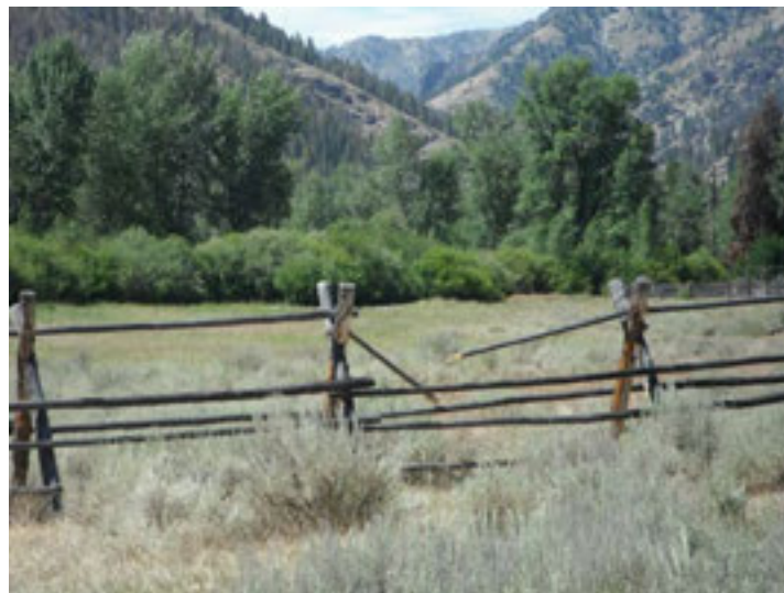
Fig. 11: Downed pole in enclosure fence. August 2, 2012.
