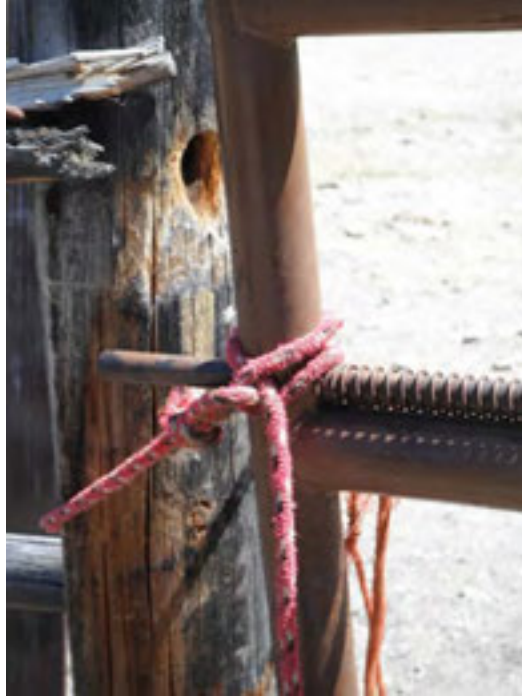
Fig. 3: Closure mechanism of West Fork gate. August 11, 2012.
