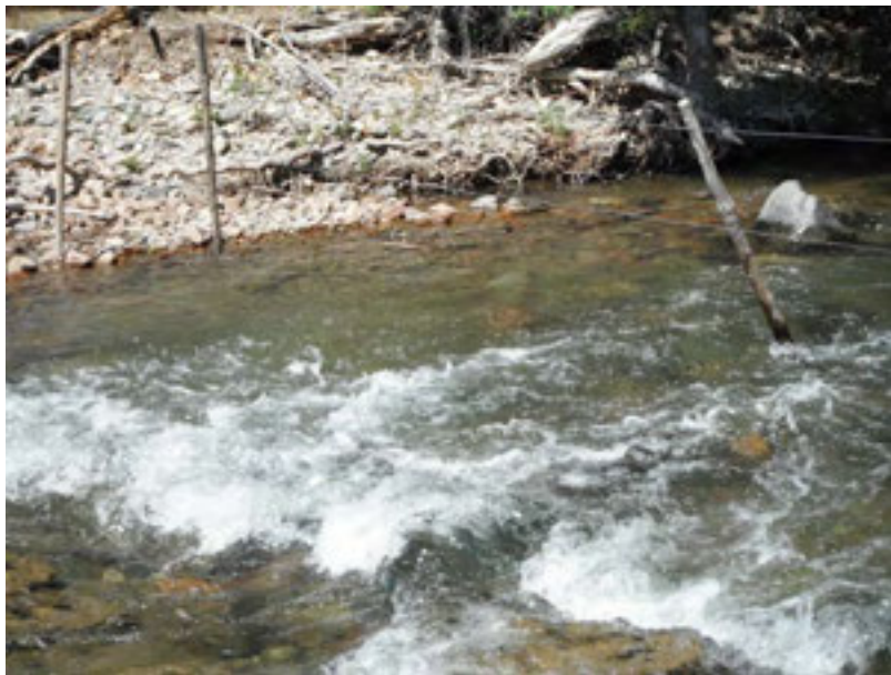
Fig. 5: West Fork ford fence, downstream side of ford, bottom wire missing. August 11, 2012.
