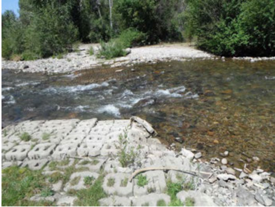
Fig. 26: Camas Creek ford #3 (near confluence with Castle Creek). Traffic drives on right side of photo, not on the pavers. August 11, 2012.
