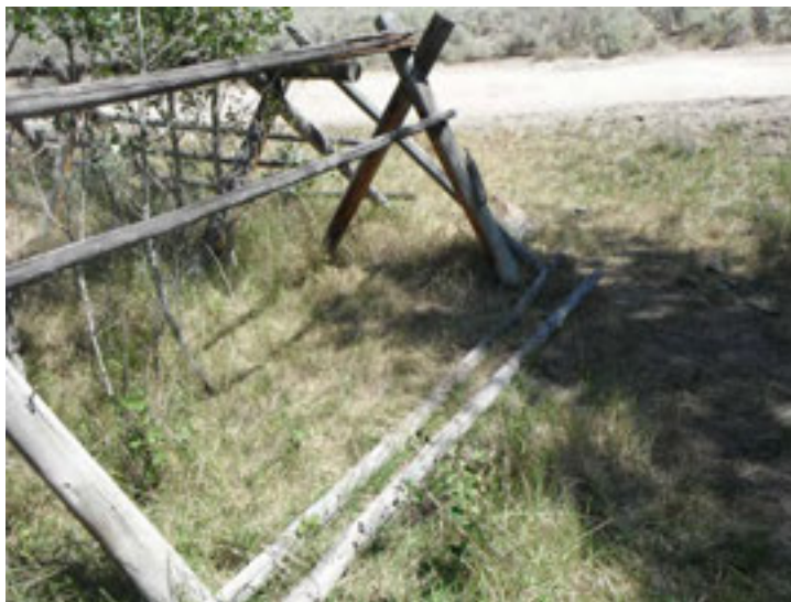
Fig. 12: Downed pole in exclosure fence. August 2, 2012.
