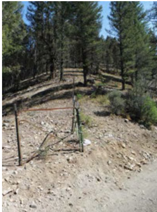
Fig. 52: Cow prints and eroding side-slope from hoof shear on road above Camas Creek fence at Furnace Creek. August 17, 2012.
